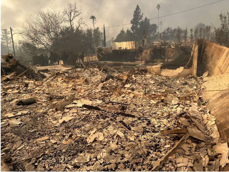
11 12 13 14 15 16 17 18 19 20 21 22 23 The burned remains of TARA’s home after the Eaton Fire.
