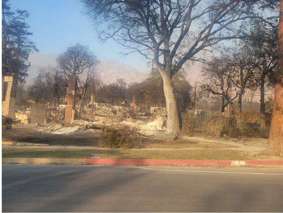
15 The burned remains of SARAH's home after the Eaton Fire.
