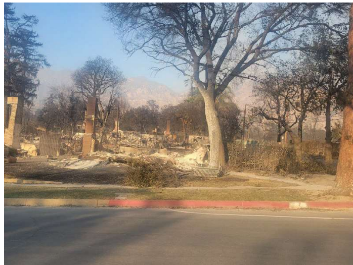
The burned remains of SARAH's home after the Eaton Fire.
